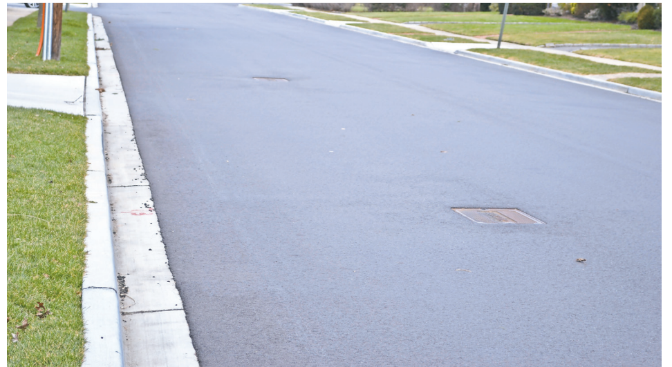
Pictured is the new roadway on Earle Avenue.
